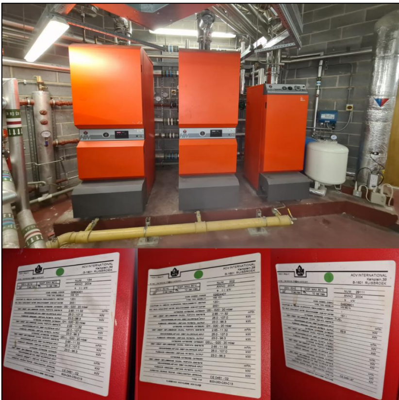
Figure 6: A good example of boiler plant in situ (top), also showing examples of the name plates of these boilers, clearly illustrating the year of manufacture, in this example 2004 (bottom).
